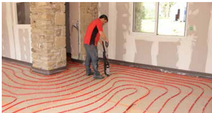
Plancher chauffant
